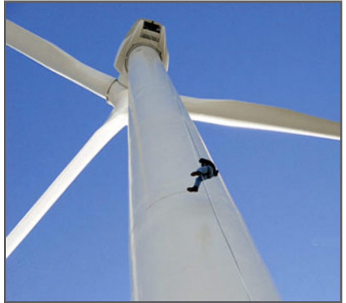
Wind turbine technicians work on towers and platforms 260-plus feet above the ground.
